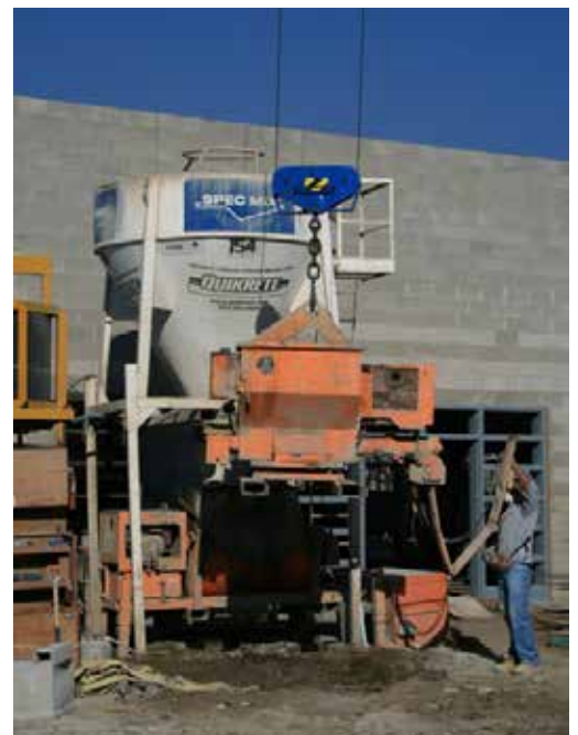
Grout Hog crane bale system in use.
